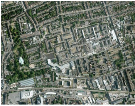
B Large post-war housing estate in Hackney
