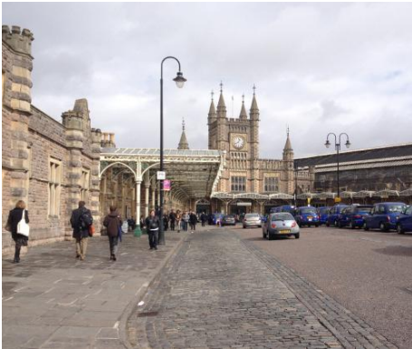
A Bristol Temple Meads Station Approach.
